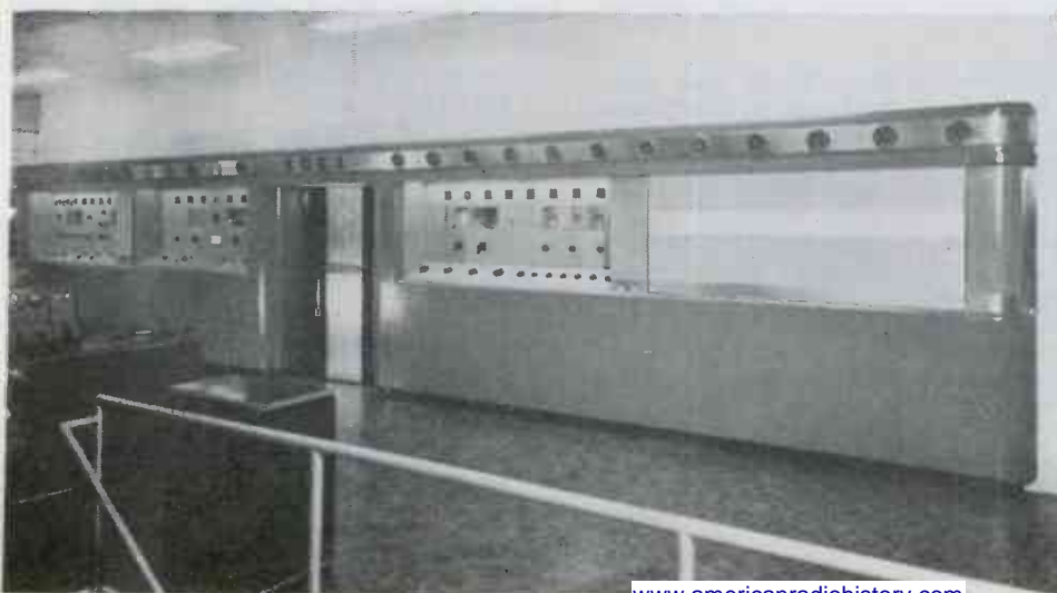
Fig. 3—This general view of KGEX transmitter shows how the vertical sliding doors are raised providing complete safety for the operating personnel while the equipment is on the air
