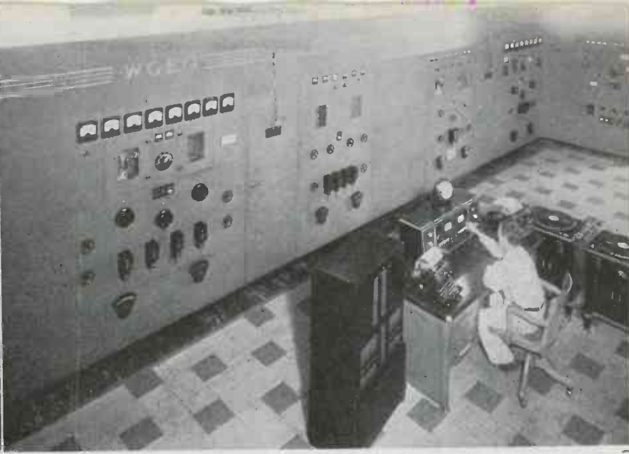
Fig. 9—General view of the main short wave transmitter room at the South Schenectady station with the 100 KW transmitter WGEX at the left and WGEX, rated at 50 KW output, at the right
